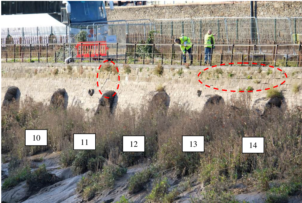
Photo 01 – Buttress B10 to B14 (Ch135m – 163m)
