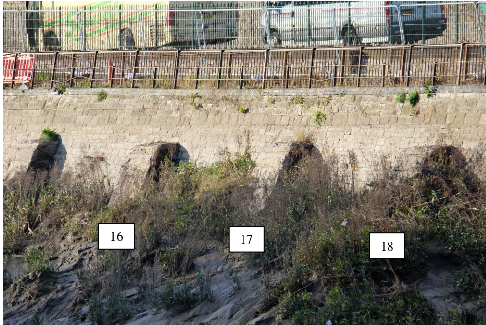
Photo 03 – Buttress B16 to B18 (Ch170m – 190m)
