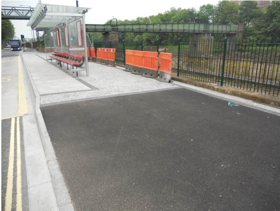
Photo 15 – Works to Cumberland Road (Ch300m)
