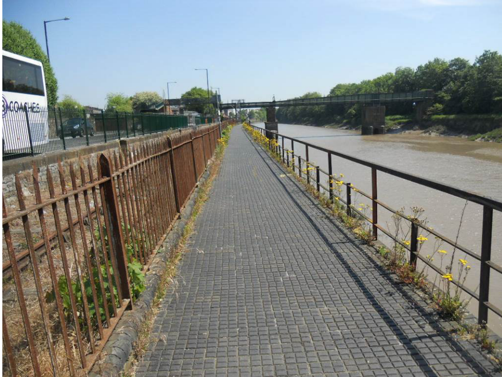
Photo 19 – General Condition of Chocolate Path (Ch215m to Ch306m)
