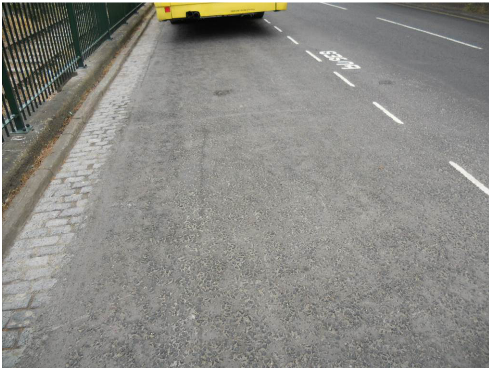
Photo 14 – Cumberland Road (Ch230m)
