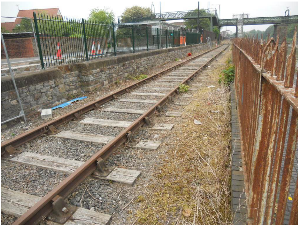
Photo 22 – Railway to the East of the Slip (Ch147m – 306m)
