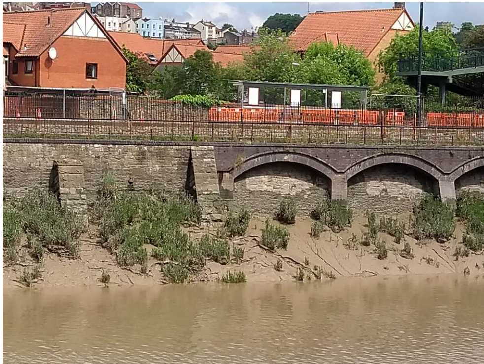
Photo 04 – Retaining Wall (Ch 285m – 298m)
