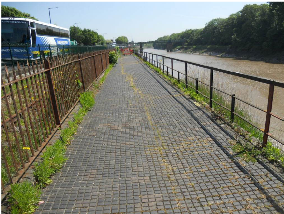
Photo 16 – General Condition of Chocolate Path (Ch81m to Ch130m)
