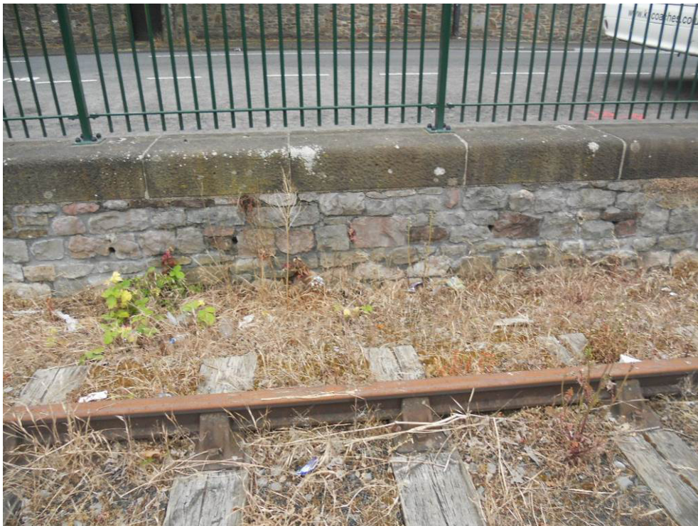
Photo 24 - Highway Retaining Wall
