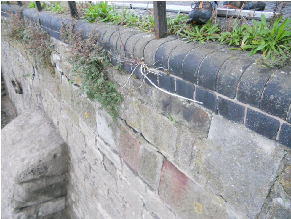
Photo 06 – Wall Near to Buttress B11 (Ch145m)
